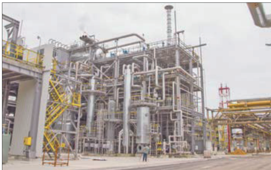
Construction and installation works at the M-450/A-135 production complex are complete.
