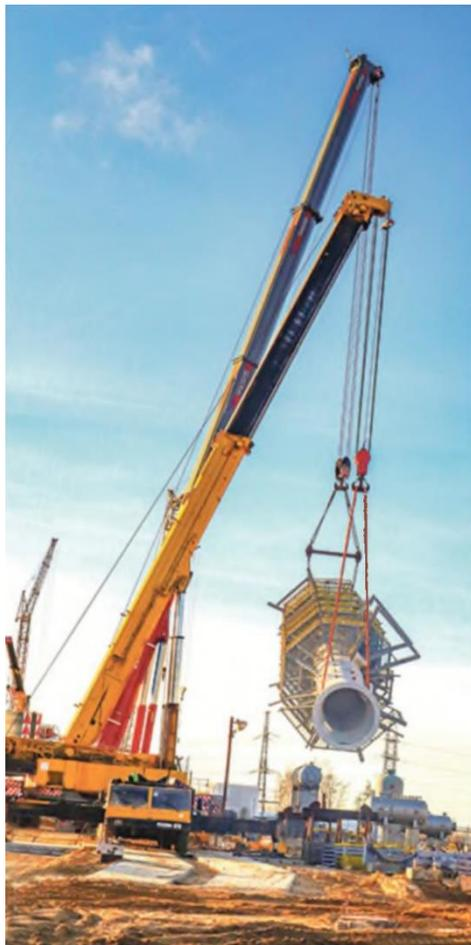
**The main manufacturing equipment is being mounted at the Methanol-500 unit.**
